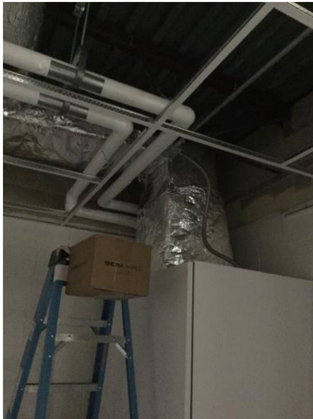
Vertical Unit Ventilator Ducted and Hydronics Piped Phase IV March 6, 2017
