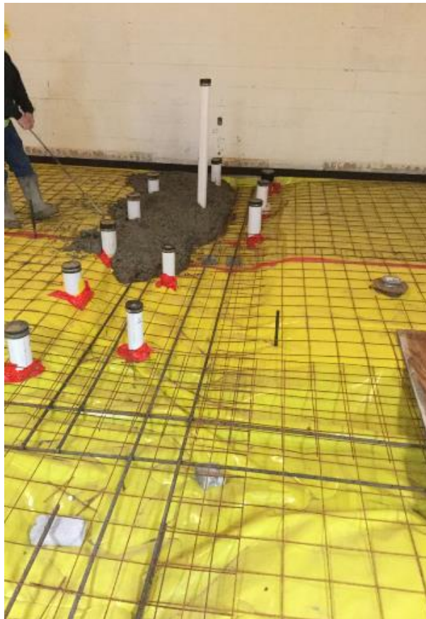
Restroomm Underground Utilities Stubbed up and Concrete Pour March 6, 2017
