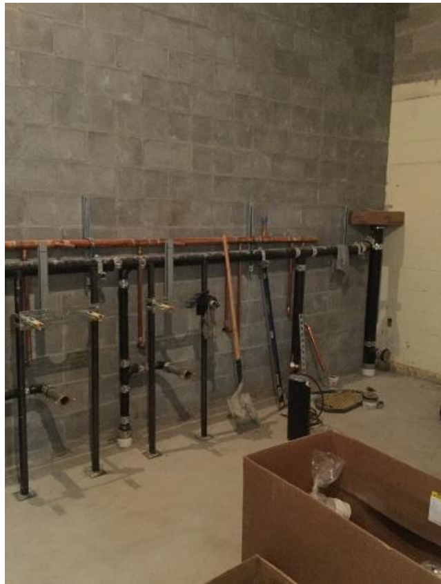
Restroom Chase Plumbing March 13, 2017
